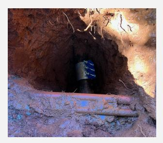
At the start of November, a tree service company noticed a small leak along Foresthill Road above the treatment plant and notified our operators. Repairs were scheduled for November 7<sup>th</sup> and completed in a couple of hours. This was a pinhole sized leak on a 6" steel line which was approximately 4 feet below grade to the top of the water main. Operators coordinated with the tree crew who already had traffic control set up at the location for a quicker repair.
