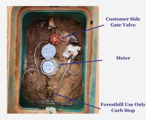
A Gate Valve, also known as a shutoff valve, is a valve located on the customer's side of the meter that allows the customer to shut their water off at any time without having district personnel present. This valve is very helpful if you ever have a leak and need to make repairs.
