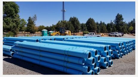
Approximately 7,000 feet of the pipeline will be replaced from the old Sebastian building to Thomas Street. Thanks to the \$700 thousand dollar water transfer and a PCWA grant, no new or additional debt will be necessary to complete this project. This section of the pipeline dates to the 1950s and has reached the end of its service life. By replacing it, Foresthill will have improved fire protection.
